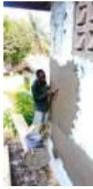
With a scalpel built, exterior plastering began.
